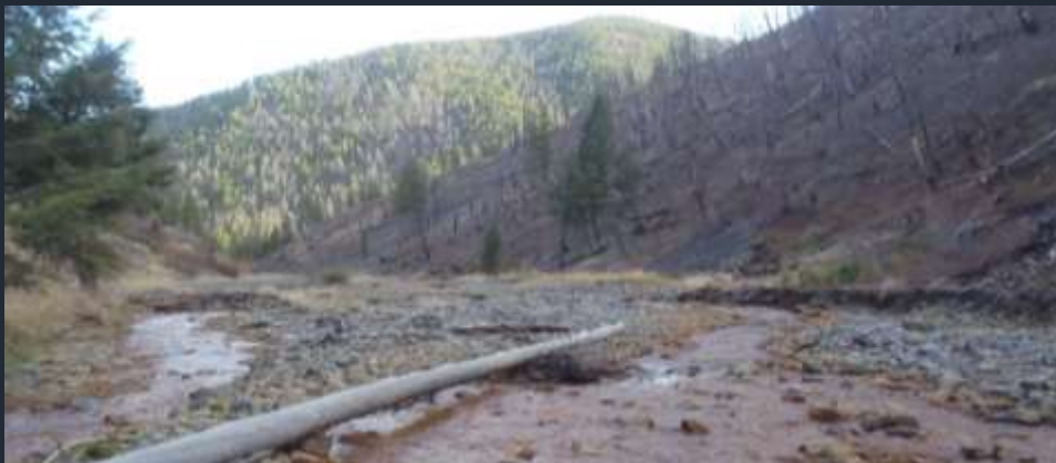
Pre in-stream stabilization (2009)
