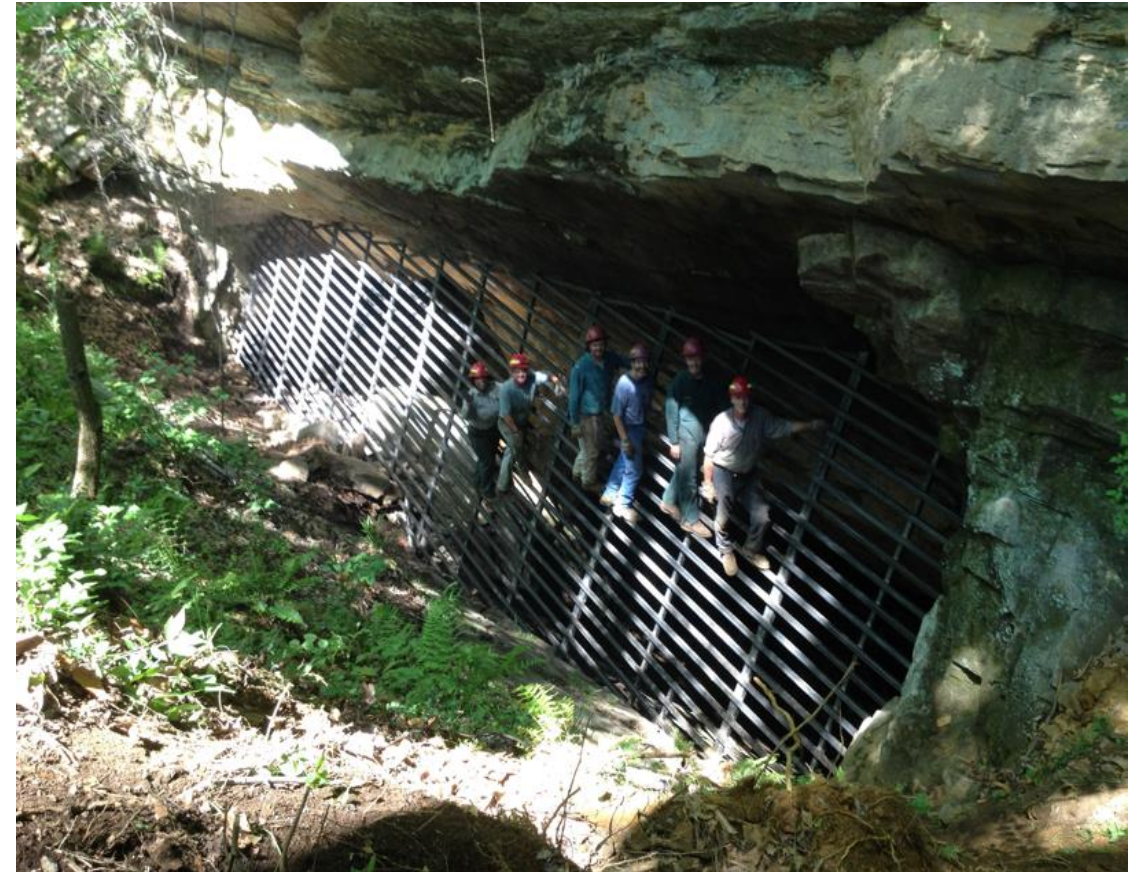
Bat gate installed on the George Washington – Jefferson National Forest
